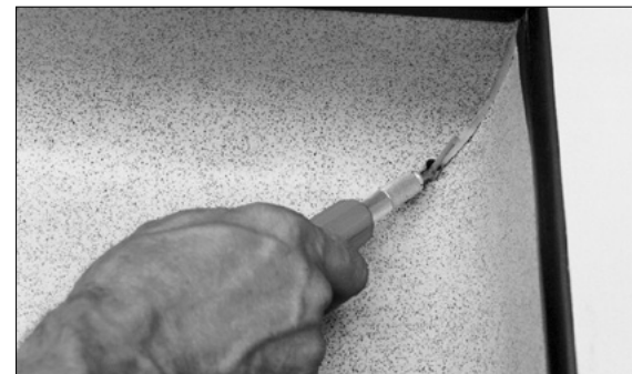
2. The X-ACTO small round router blade should be used for trimming the cooled weldrod on internal corners.
