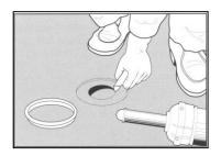
Around flush drain openings, heat the sheet and mark the location of the drain using a clamp ring. Then cut a small hole in the centre of the drain within the mark. Heat the flooring and press the clamp ring down into the edge of the drain. When using an adjustable clamp ring, make sure it fits tightly. Trim the material around the perimeter of the ring.
